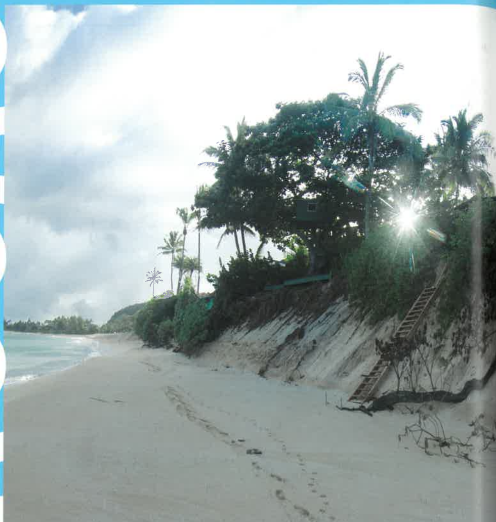
Erosion affects houses on the North Shore
